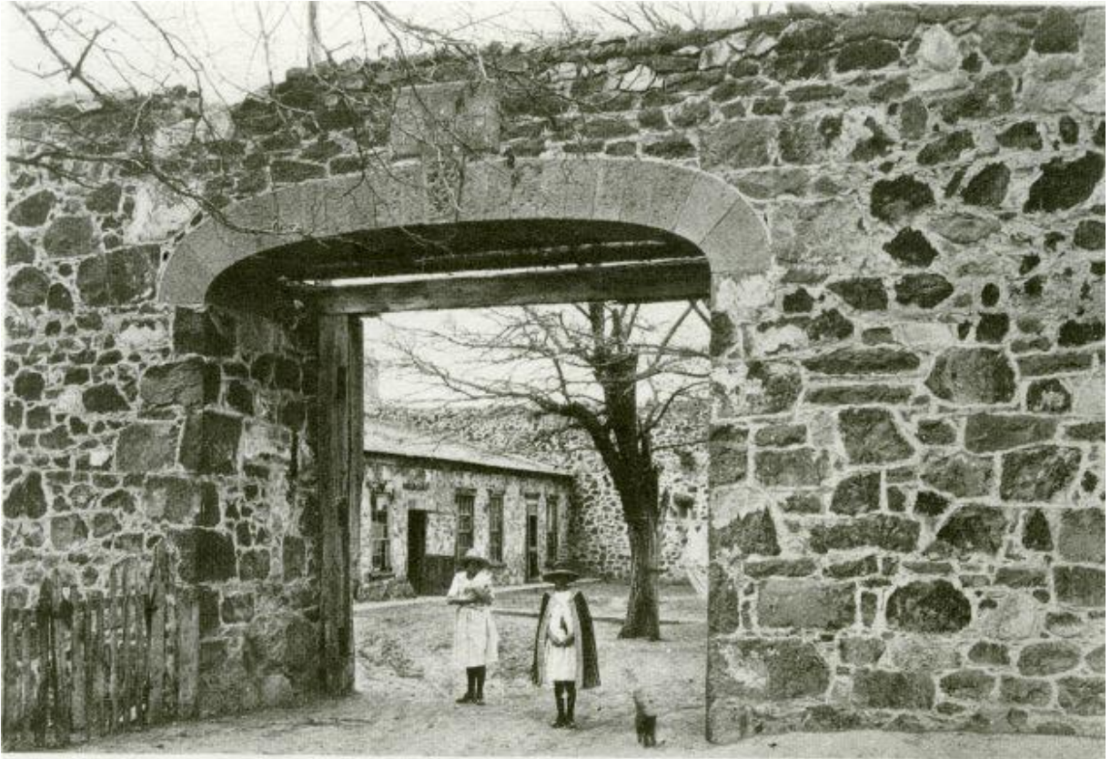
ENTRANCE TO OLD COVE FORT, SOUTHERN UTAH.
